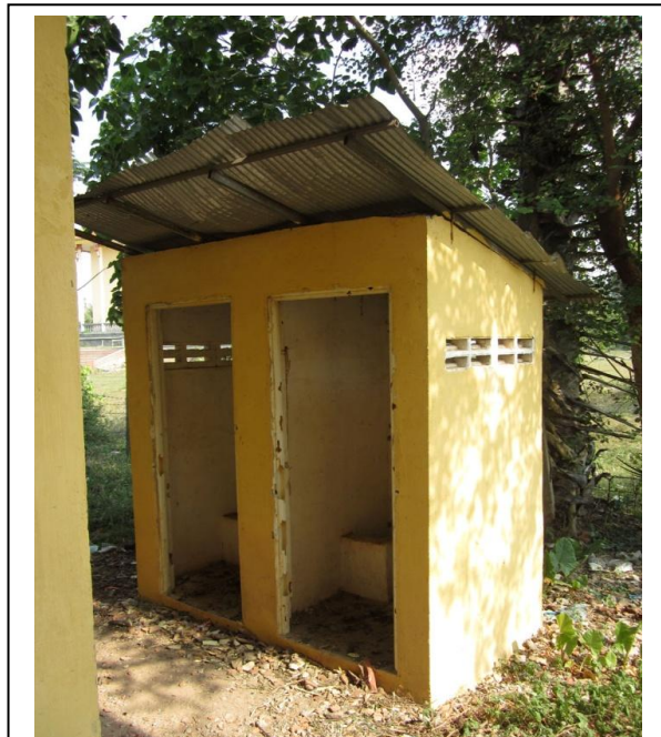
Bathroom before repairing.
