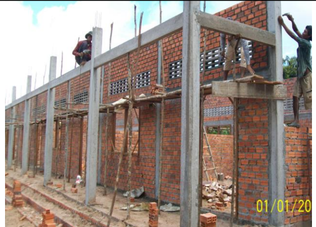
Colin M.Davis school was under construction
